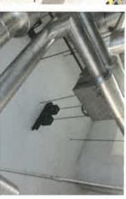
Above and right: Plant in the landlord's lower basement plantroom is mounted on anti-vibration mountings
